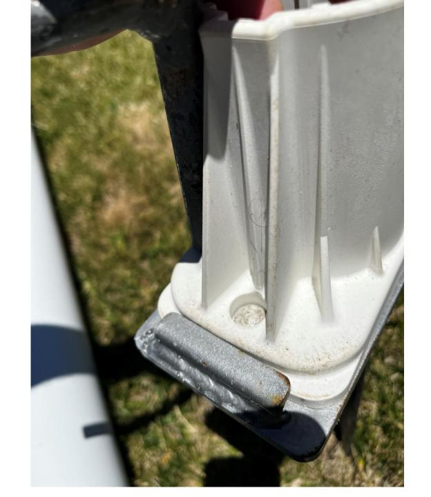
Place post into ground plate ready to lift rail onto posts.
