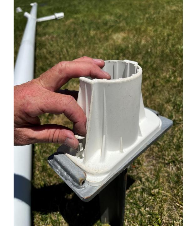
Use the Barriers tool to secure the PVC rivet to the ground plate.
