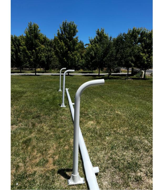
The rail can be used as your line. Place the ground plate in the correct position.
