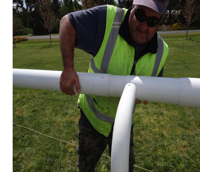
Ensure the join remains inside the tee at the post.
