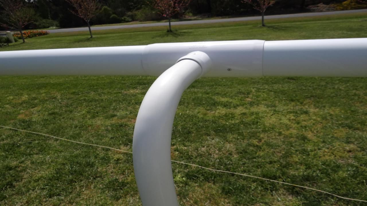
One length of rail. The next piece of rail slides over the insert on the left.
