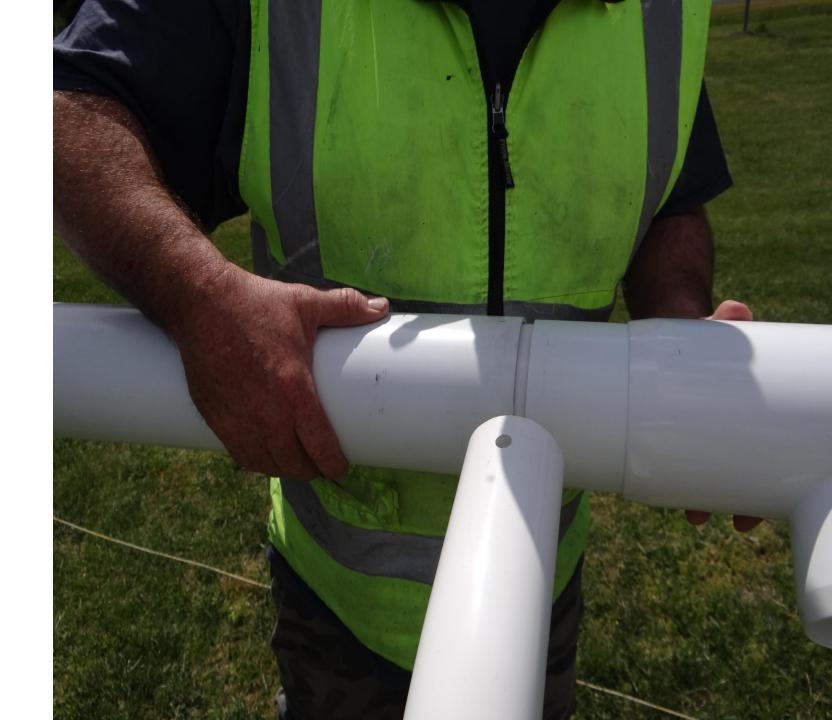
If the glue from the insert becomes unsecure. Drill a hole and use a pop rivet to secure the insert inside the rail. 400mm exposed, 200mm inside the rail.
