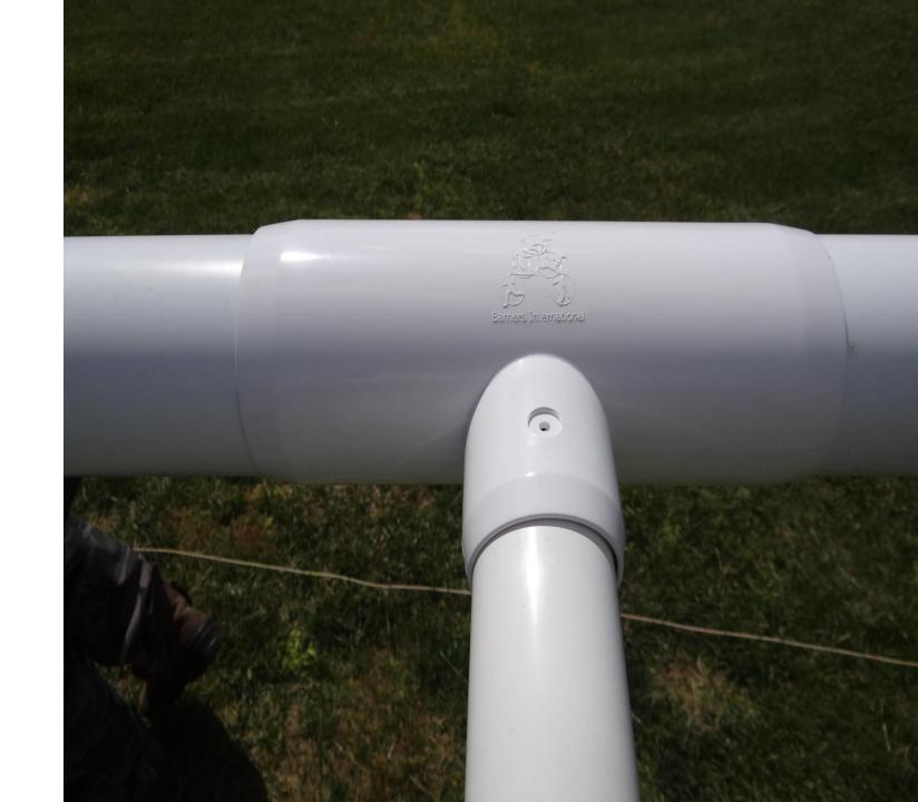
Drill hole at top of tee at pre-drilled hole in tee and through top of post only.
