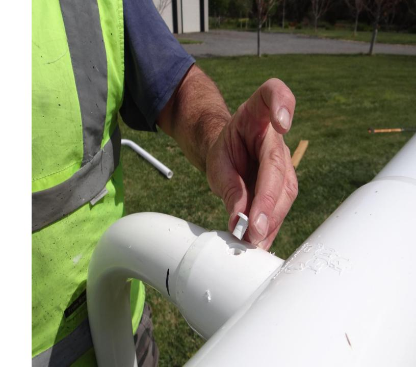
Use rubber mallet to hammer PVC rivet into hole.
