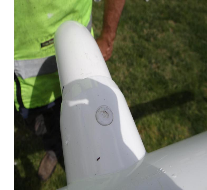
Secure the rail and tee at only one tee per length of rail and not on an end. This stops the rail sliding.
