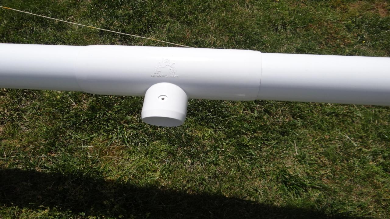
Lift the rail onto the post. This is how the first post should look.
