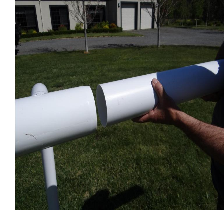
Drill a hole through top and bottom of tee and rail. Use red pins to secure rail inside the tee. This should be repeated at a second tee. Then remove one tee and the piece of rail is easily removed and easily re-installed.
