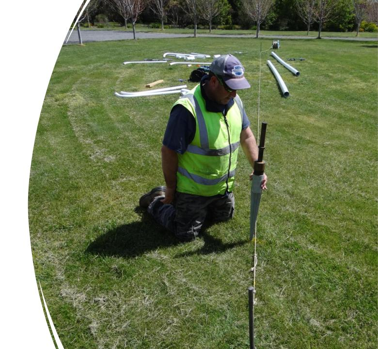
The ground fixings should be installed consistently at the same height to the rope line.
