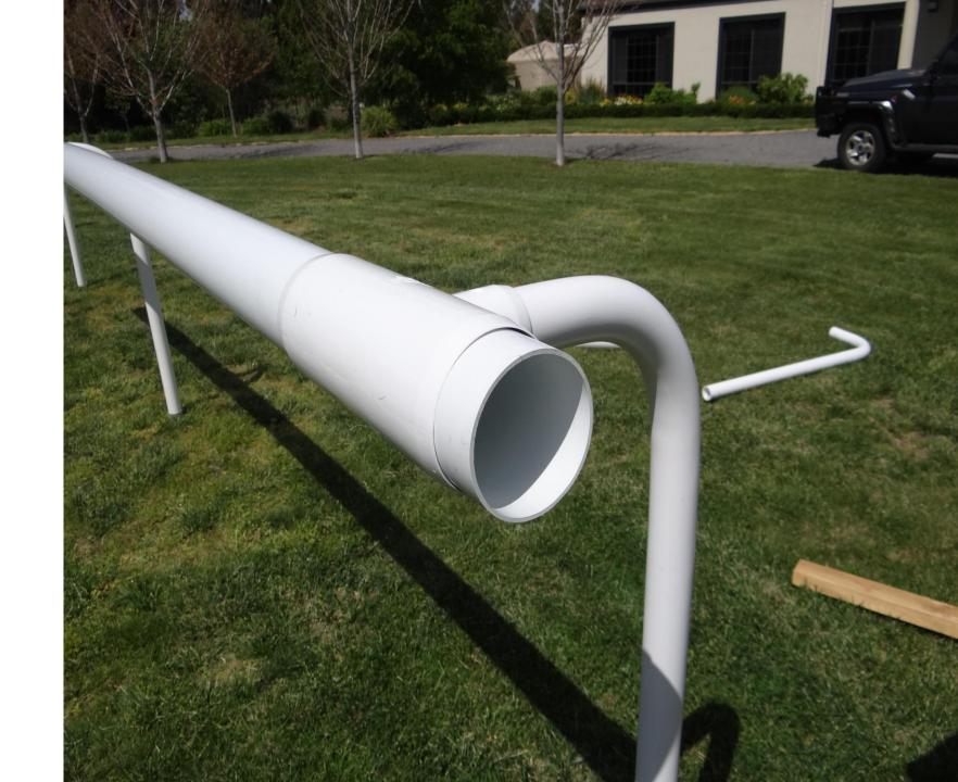
The rail join. The rail slides over the insert from the previous rail.
