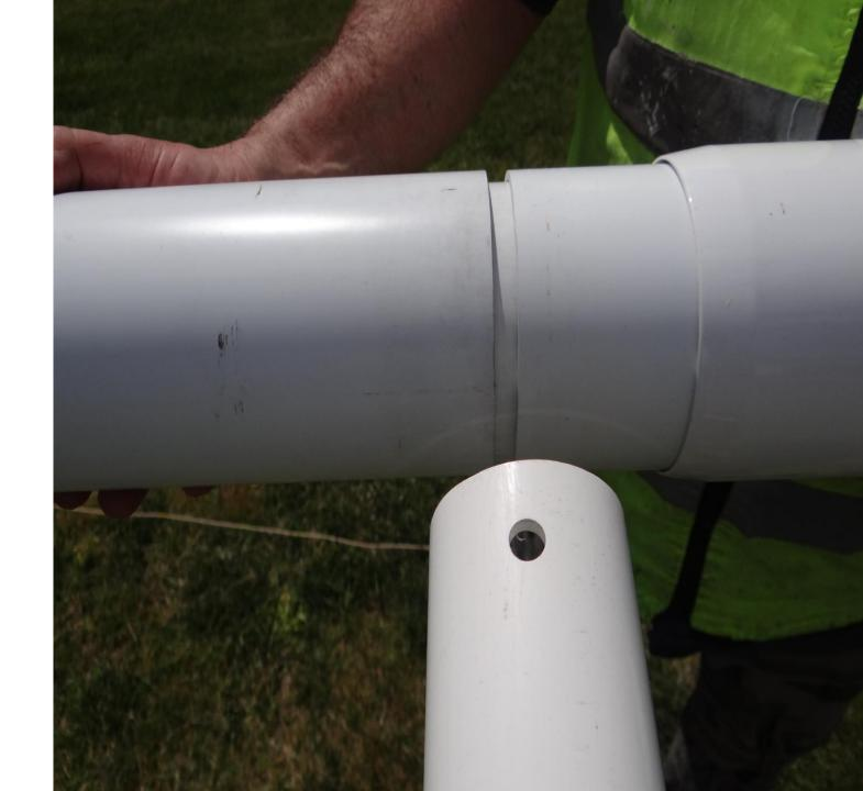
Securing the tee. Push post hard into tee.
