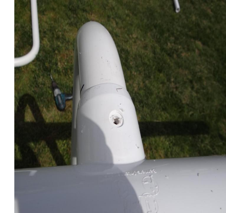
Put PVC Rivet into hole to secure tee and post.
